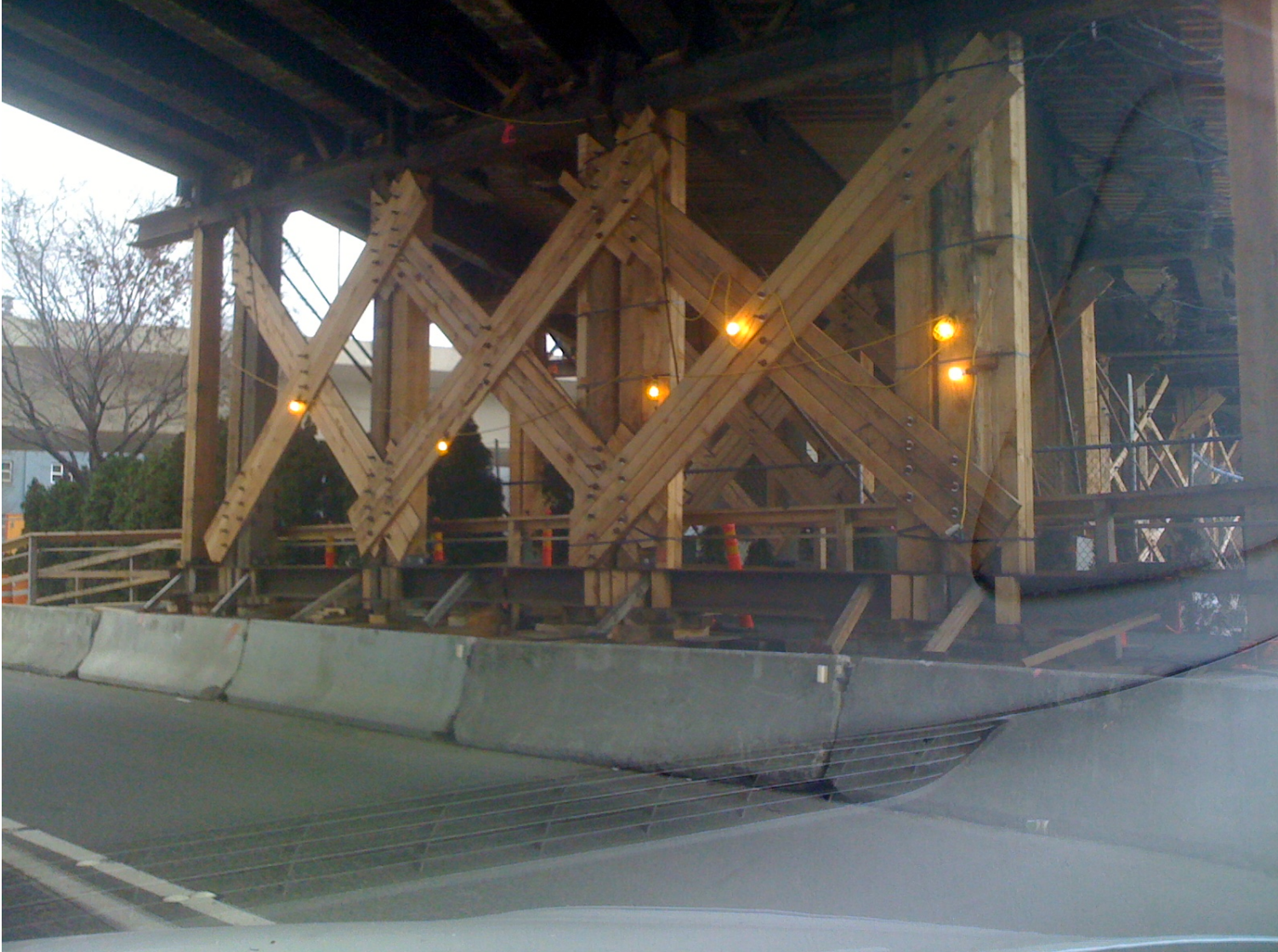
As seen at this road construction project underneath the Spokane Street Freeway.
