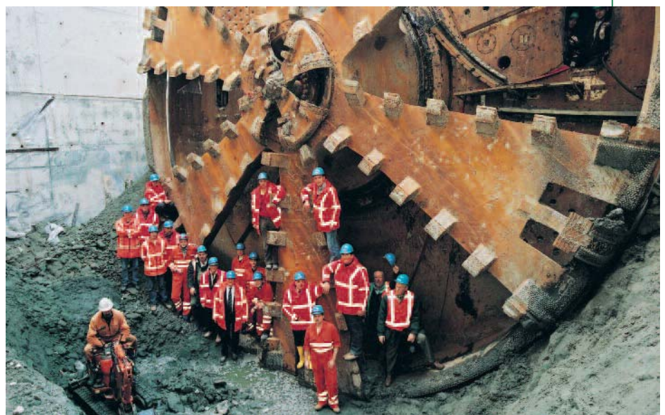
Below: Breakthrough of the Westerschelde machine, in The Netherlands
